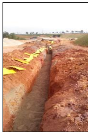
Laying of fine Sand (covering the gas pipe)
