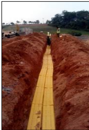
Laying of Protection Cover for gas pipe
