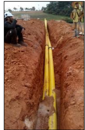
Laying of Gas Pipe
